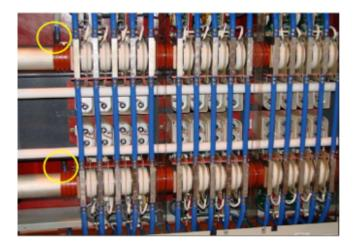
Figure 1: Load bridge water-cooled bus ends with SCRs and capacitor installed (2 out of 6 visible)
