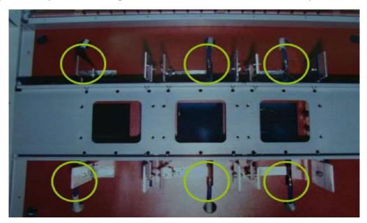
Figure 2: 6 pulse Load bridge water-cooled bus ends without SCR and Capacitor installed
