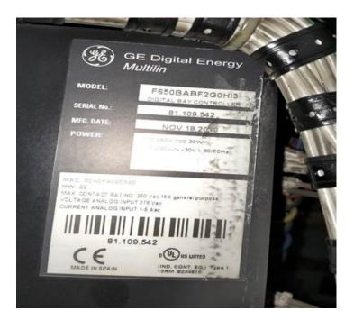
2. GE Multilin 650 Relay for Line Incomer Protection ( 6.6KV MV System) Protection Against: IDMT INSTANTENEOUS OVER CURRENT/EARTH FAULT (50/51/50N/99) Required Quantity:05nos
