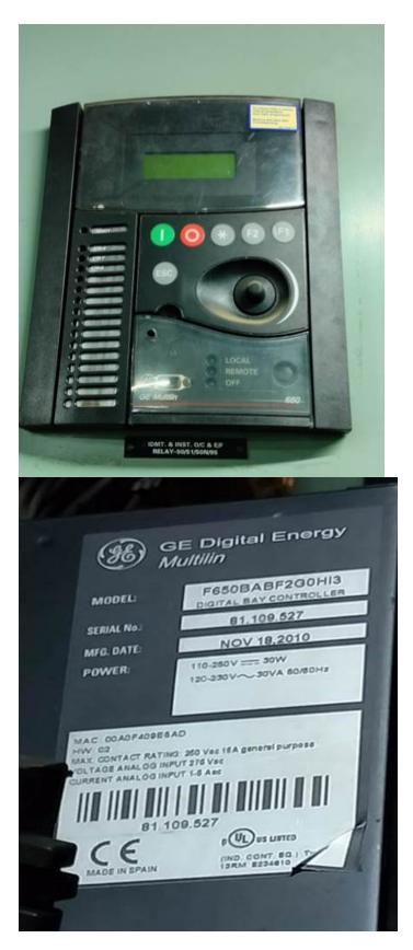
**4.** GE Multilin 650 Relay for Motor Differential Protection ( 6.6KV MV System) Protection Against: MOTOR DIFFERENTIAL (87) Fault Only for Motor feeders above 1000KW.
