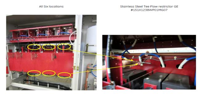
2. Load bridge rear view and locations of 6 stainless steel 'Straight flow restrictors'
