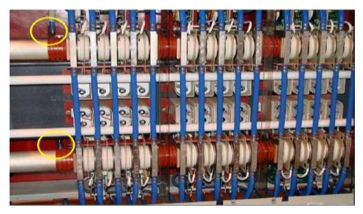
Figure 1: 6 pulse Load bridge water-cooled bus ends with SCR and Capacitor installed
